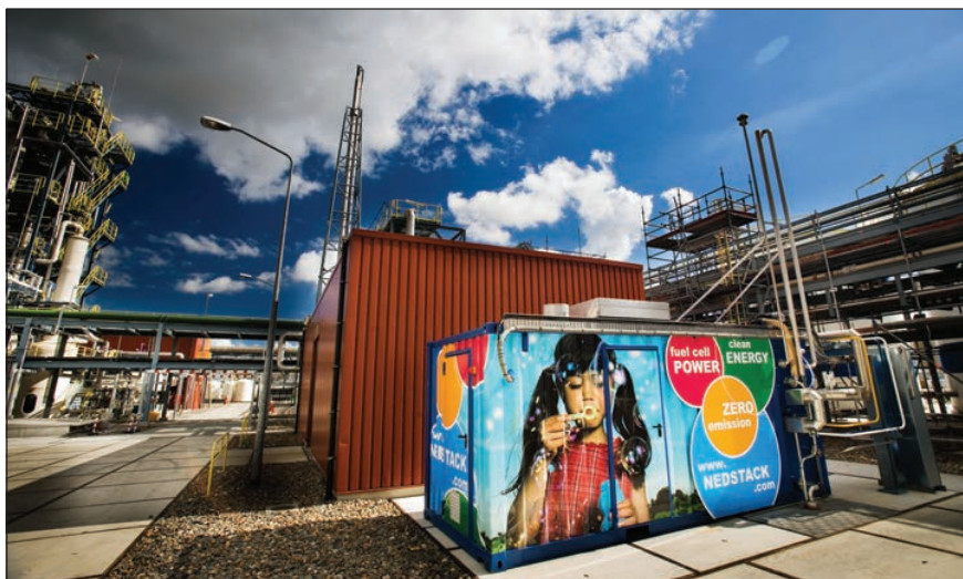
Nedstack owns a 70 kW PEMFC power plant at a chlor-alkali factory in Delfzijl, The Netherlands, with no major system components replaced since the start of operation in 2007.
